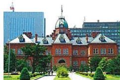
Former Hokkaido Government Building (Red Brick, Akarenga)
